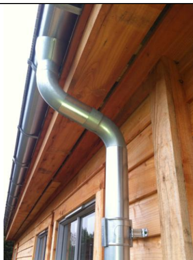
Fig 2 Proposed timber cladding + rainwater goods
